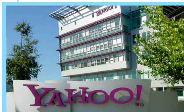
Yahoo! Corporate Headquarters, located on 34 acres in Sunnyvale, California, installed 19 Code Blue units throughout their extensive campus and parking facilities.
