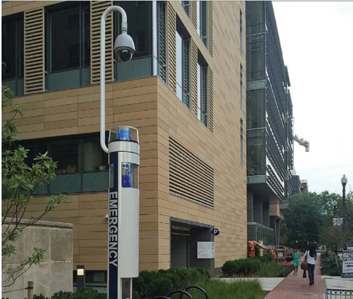
A Code Blue Emergency Light Tower, located on the Washington University Campus.
