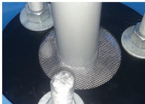
**\*For an extra-strong seal, a bead of silicone caulk can be put on the gasket from bolt hole to bolt hole before setting the gasket into place and around the conduit.**
