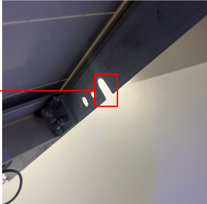
Cellular Antenna Install Location
